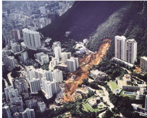
Po Shan Road Landslide, Hong Kong, 18.06.1972, www.hkss.cedd.gov.hk
