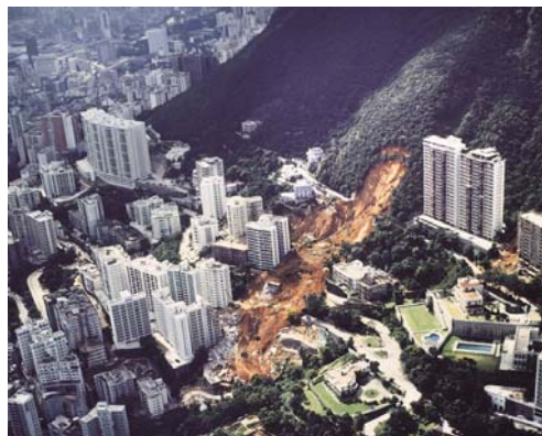
Po Shan Road Landslide, Hong Kong, 18.06.1972, www.hkss.cedd.gov.hk
