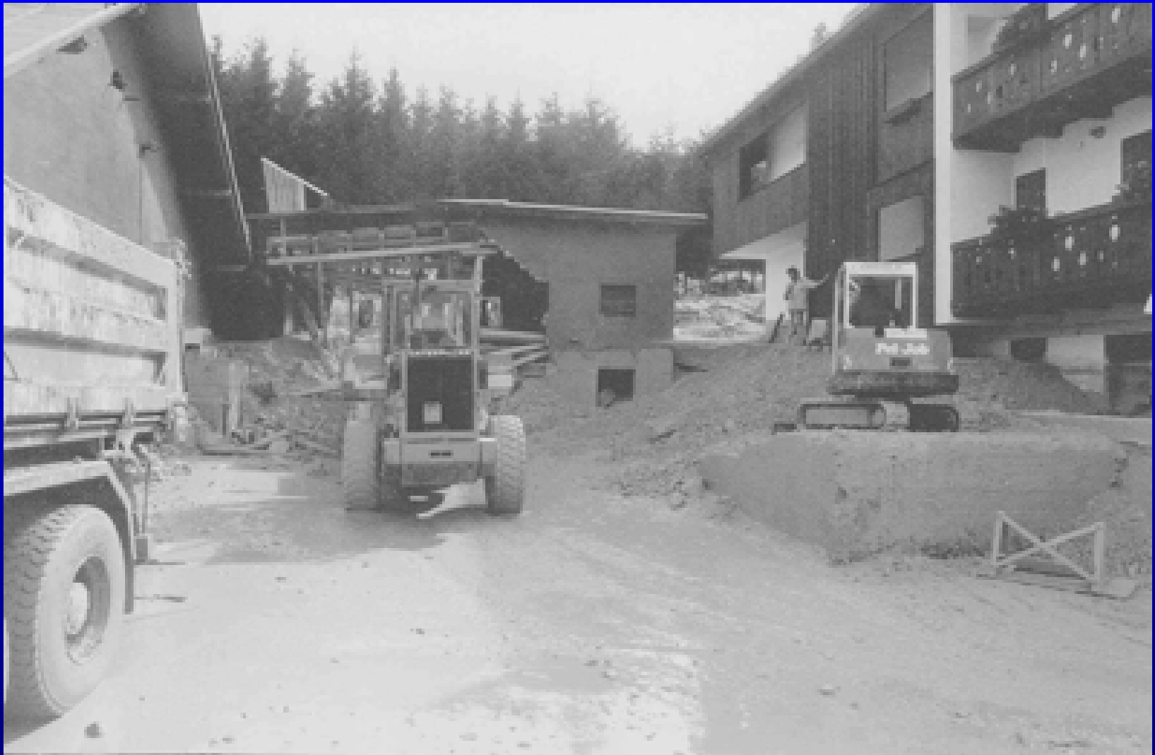
Demolished building due to load on the roof due to the flow (Photo: Zanfron)
