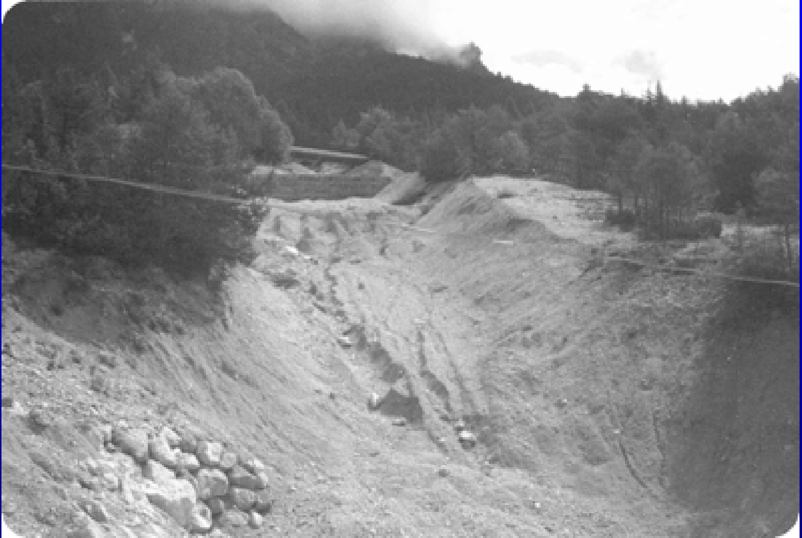
Downstream retention tank at 1010 m
